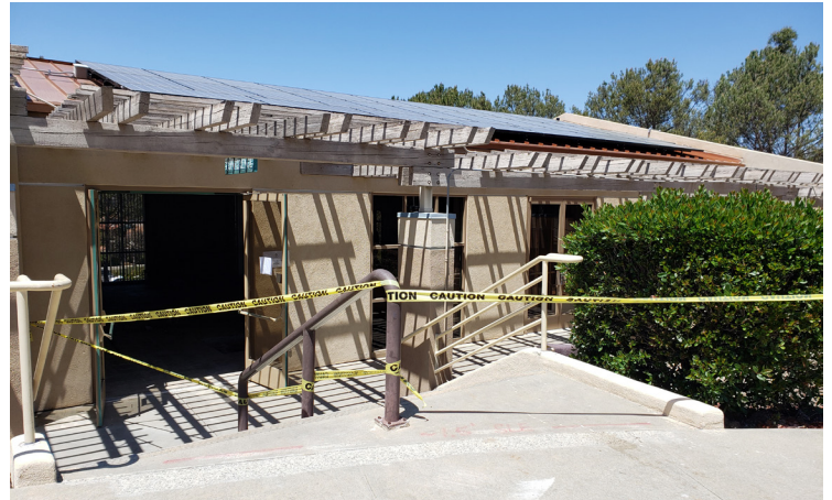
Limited access to the staircase from the upper parking area.
